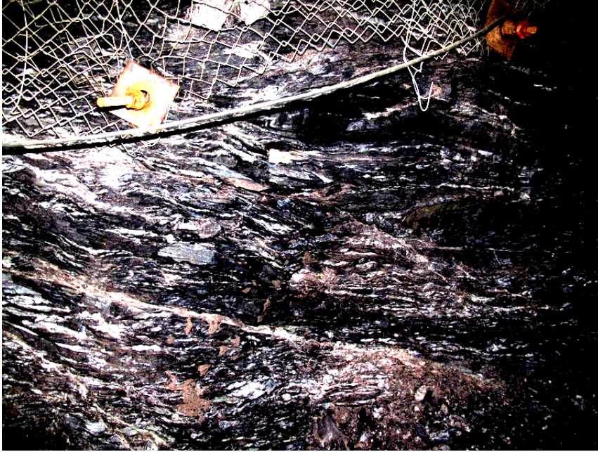
Fig. 6 Illustration of the deformation intensity in the north side of crosscut V1-XXI in the stationing section 460-510 m.
