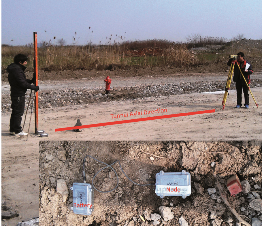
Fig. 5 Deployment of sensor nodes and surroundings in the field. The MEMS sensors were deployed along with or perpendicular to the tunnel axial direction, and a total station was set for the absolute value of the settlement as a reference.
