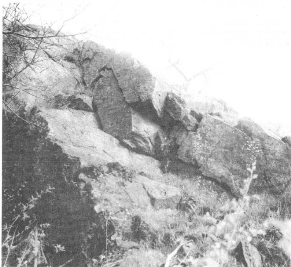
Fig. 4. Disintegration of the surface part of the slope beneath Jezerka in NW Bohemia.
