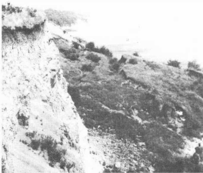
Fig. 6. Landslide in the former village of Čermníky, which took place in 1969 due to fluctuation of water level in the reservoir. Photo T. Spanilá.
