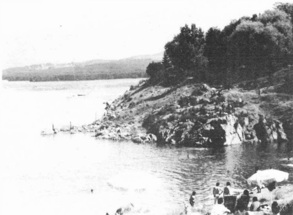
Fig. 4. Landslide due to the operation of waterwork Iskar. Photo G. Simeonova.
