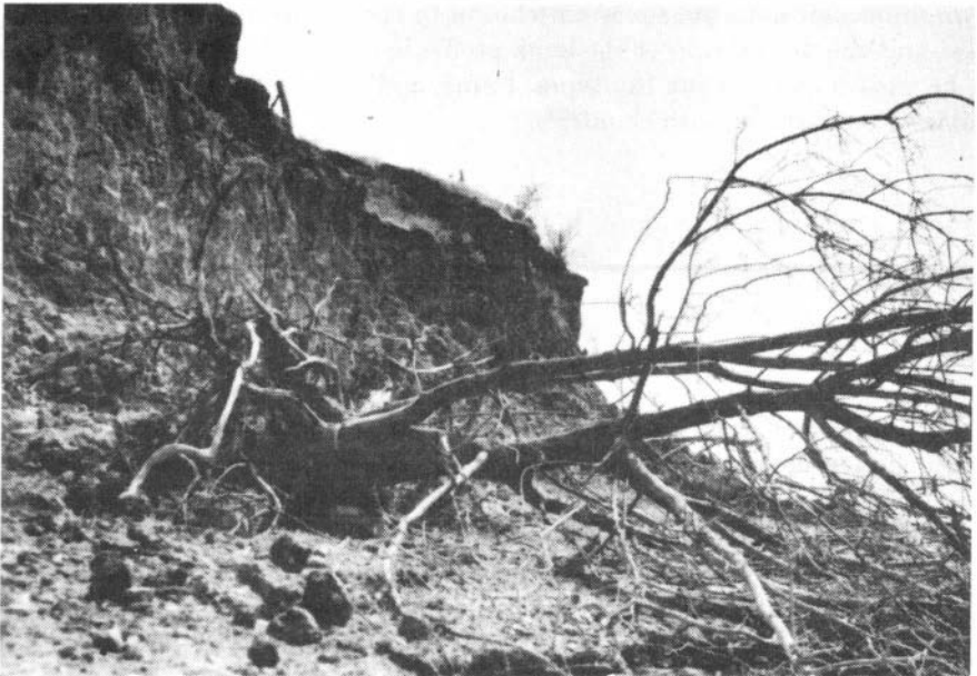
Fig. 9. Tumbling of individual blocks, dropping and breaking off of weathered clayey formations on the Nechranice waterwork. Photo T. Spanilá.
