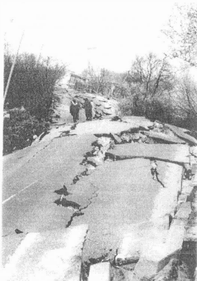
FIG. 1. Road destruction between Zlatni Piasaci and Varna near the bus station "Journalist" at the Bulgarian Black Sea coast. Landslide of April 4, 1997. Photo by G. Frangov
