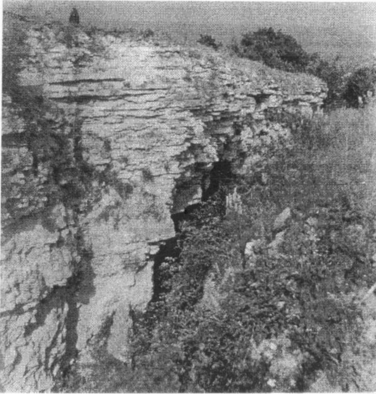
FIG. 7. The crack wall above the uppermost step of the Aladja-manastir - Zlatni Piasaci landslide. A typical example of the last stage of creep movements in a deformation described as of the blockage-consistent type - a shear plane propagating to the surface results in tensile crack formation and new step subsidence. Photo by B.Košťák
