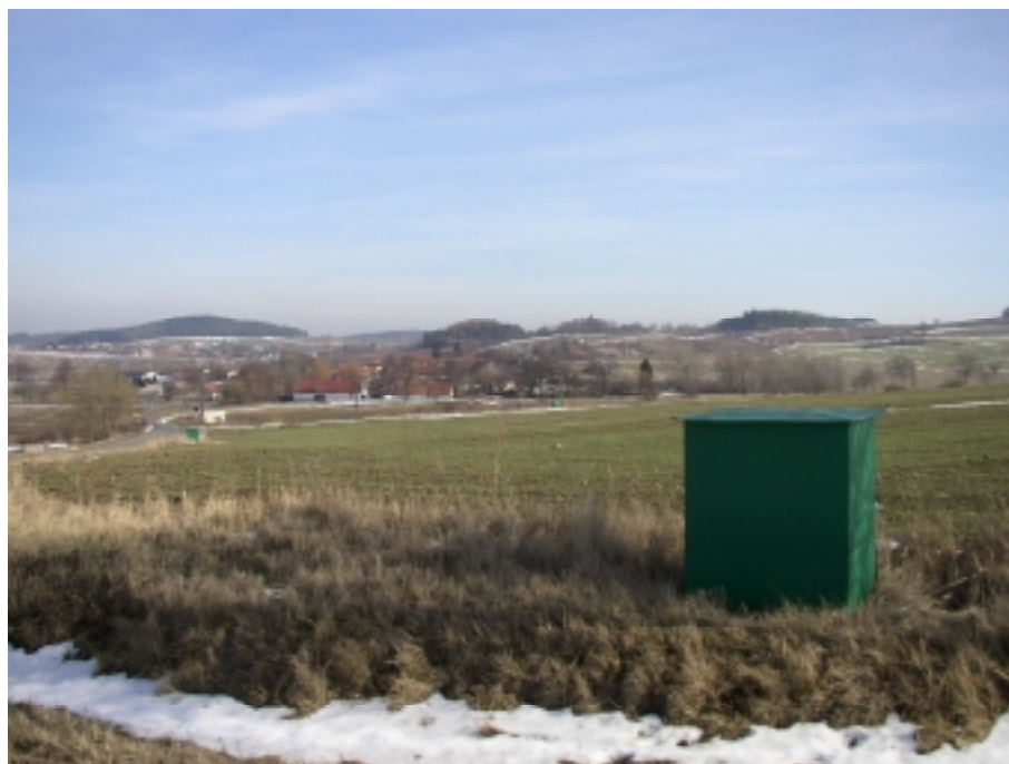
Fig. 7 Photograph of the measuring station of levelling and deep measurements
