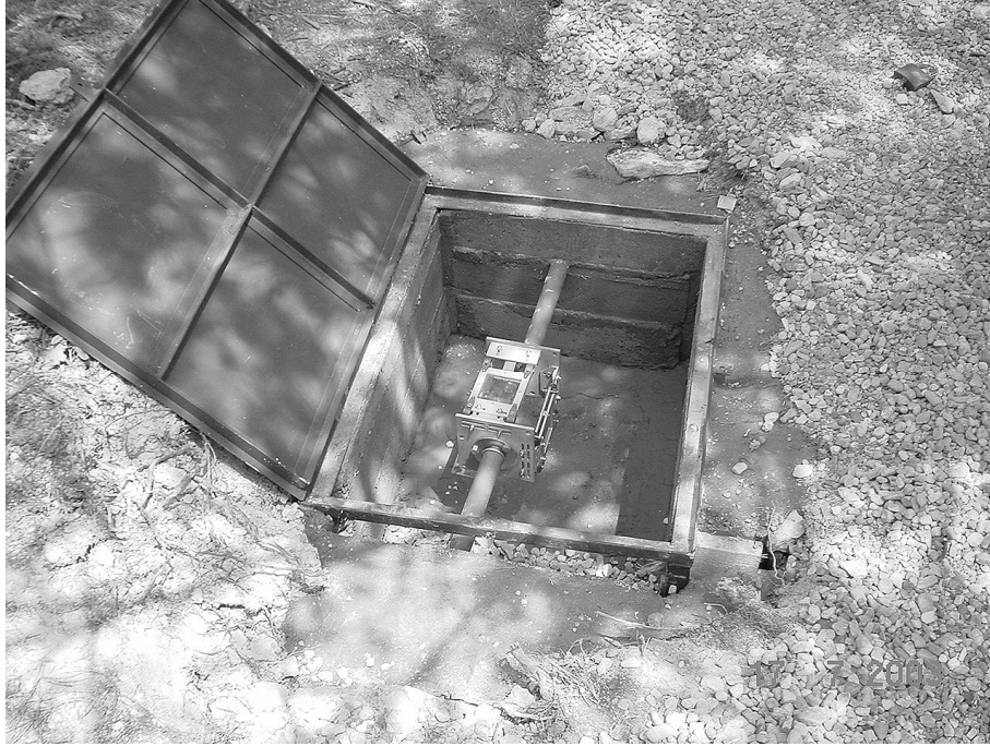
Fig. 4 View of the new monitoring site
