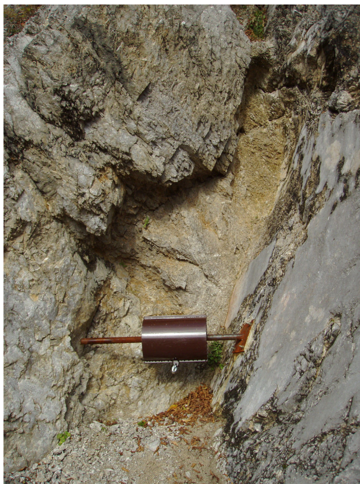
Fig. 6 Installation of TM71 crack gauge on the Raša fault in the quarry at the foot of Vremščica mountain
