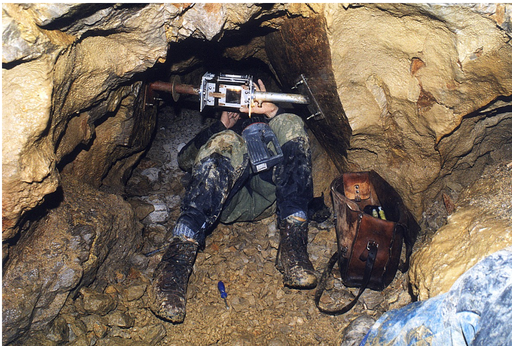
Fig. 2 TM71 device installed across the fault in Postojna cave system (Postojna 2)
