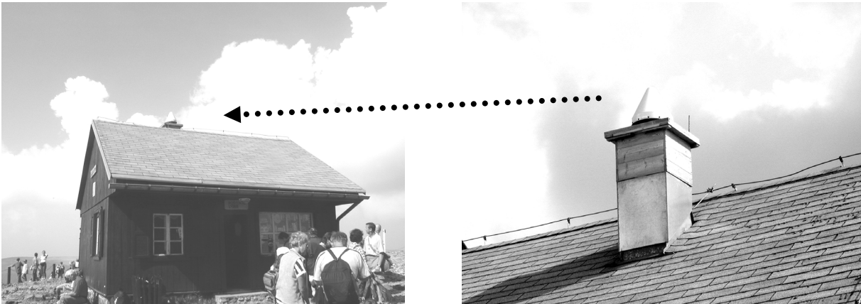
Fig. 1 Antenna position at the chimney of the Česká Poštovna building - station SNEC.
