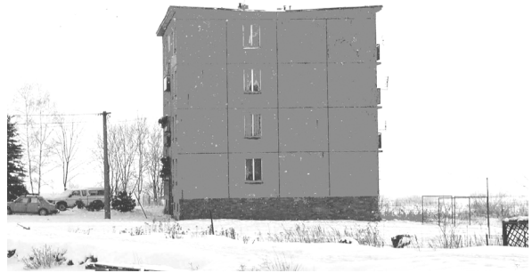
Fig. 5 The POUS permanent station
