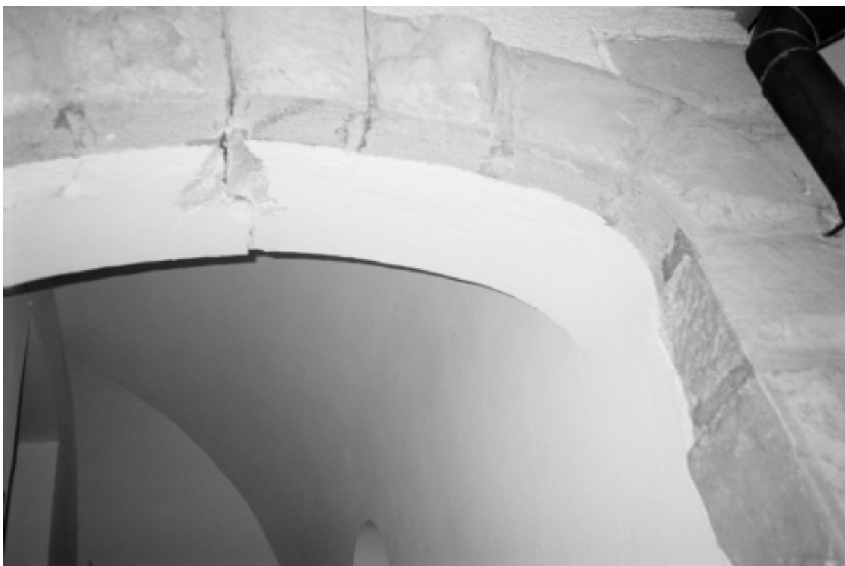
Fig. 7 Displaced vault above the church door at Miętus two.
