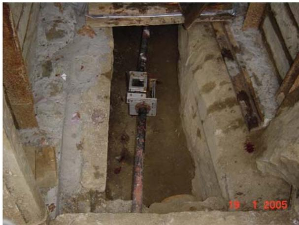
**Fig. 4** View of monitoring point 6. The left lateral displacement is obvious.
