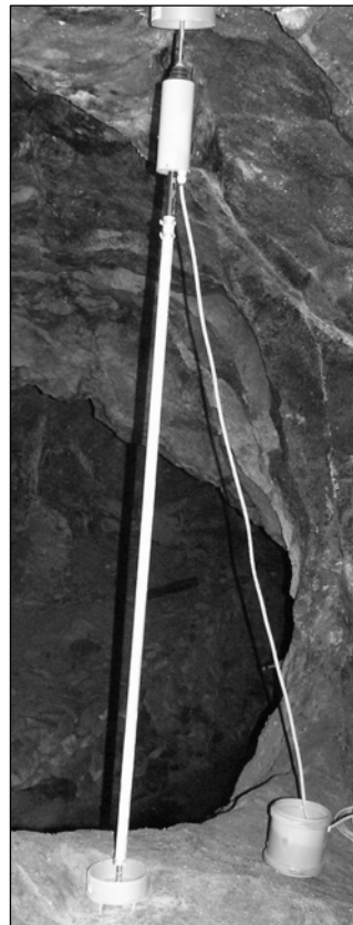
Fig. 11 Convergence meter KK1 with dismantled covering.
