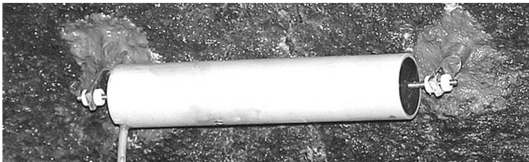
Fig. 8 Sensor for joint aperture-cased sensor HS25 installed in vertical joint (enclosure IP68). Station KD2.
