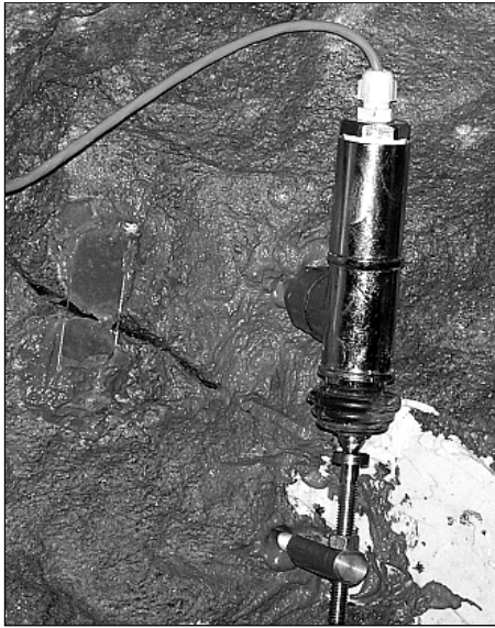
Fig. 9 Sensor for joint aperture measurement at station KD1. On the left of the sensor, a check glass slide is pasted across the joint.
