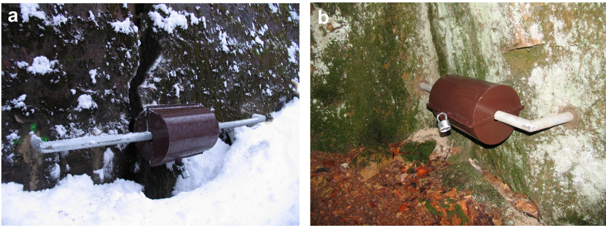
Fig. 5 Detailed location of the TM-71 crack-gauges.
