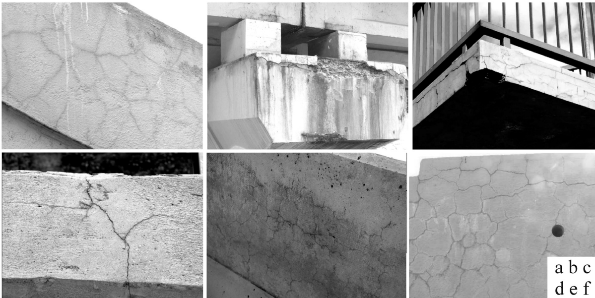
Fig. 1 Macroscopically observed ASR cracks – floor framing arch (Tuřice, part a), construction beam (Trutnov, part b), landing front (Lysá nad Labem, part c), crash barrier (Prague, parts d, e, accepted from Horský et al. 2007, modified) and face side (Dolany, part f, accepted from Míčka and Klier 2006, modified).
