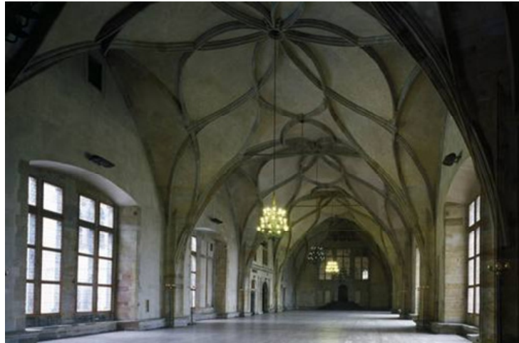
Fig. 2 Inside space of the Hall.
