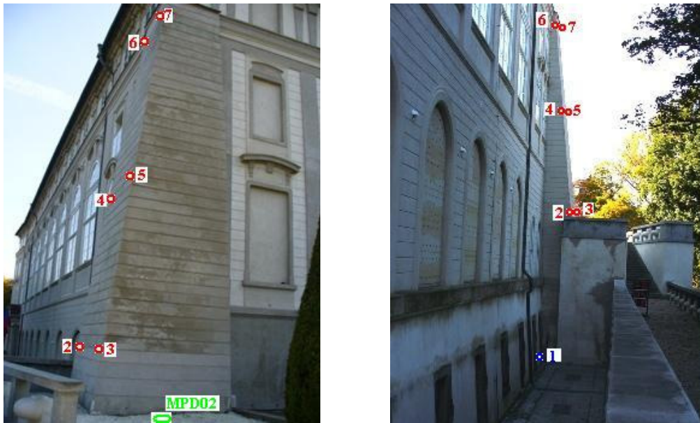
Fig. 6 Front view of Mathey buttress (in eastern direction) and side view (in western direction).
