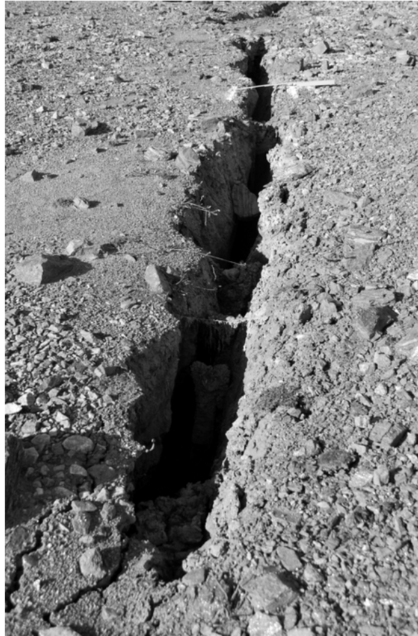
Fig. 4 View of the largest fracture (photo taken, 22.05.2009)
