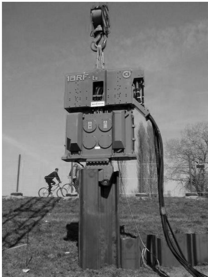
**Fig. 3** Demonstration of the overhead vibrator (photo: [www.ice-holland.com](http://www.ice-holland.com).)
