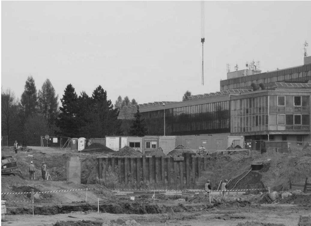
**Fig. 2** Part of sheet pile wall in the building pit (photo taken by: Lednická.).
