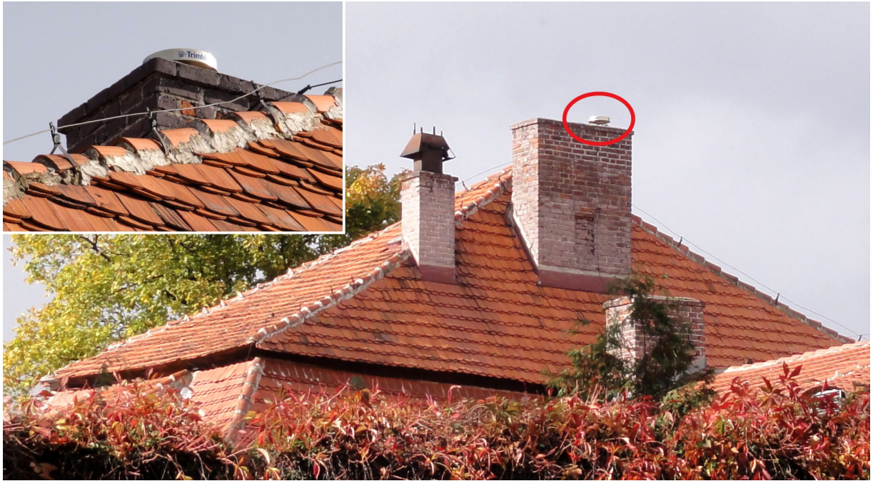
Fig. 1 GPS antenna (Trimble DM Choke-Ring (TRM29659.00 NONE) of KSIA station, mounted on the roof of the Książ Geodynamic Laboratory building.
