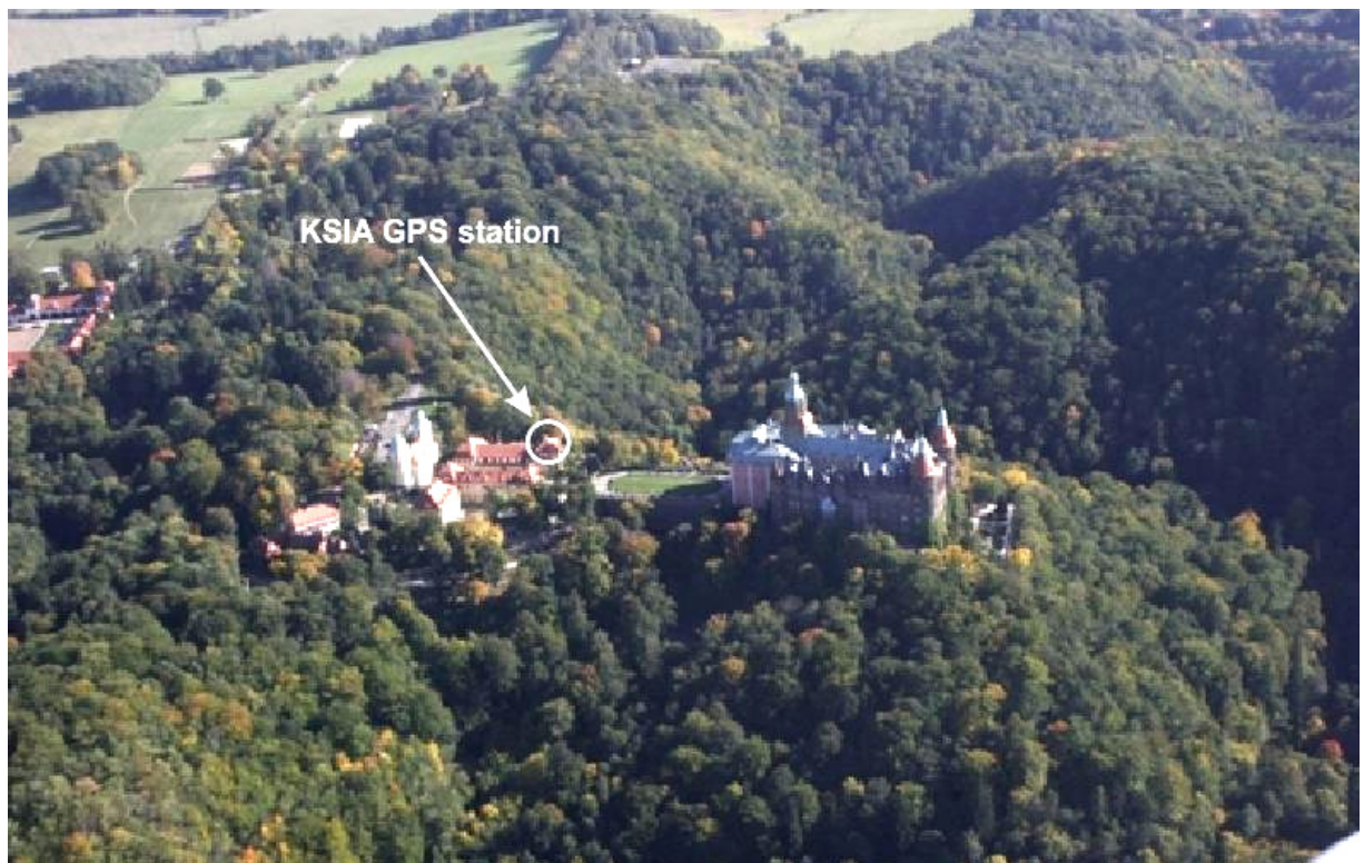
Fig. 2 GPS antenna mounted on Książ Geodynamic Laboratory building.
