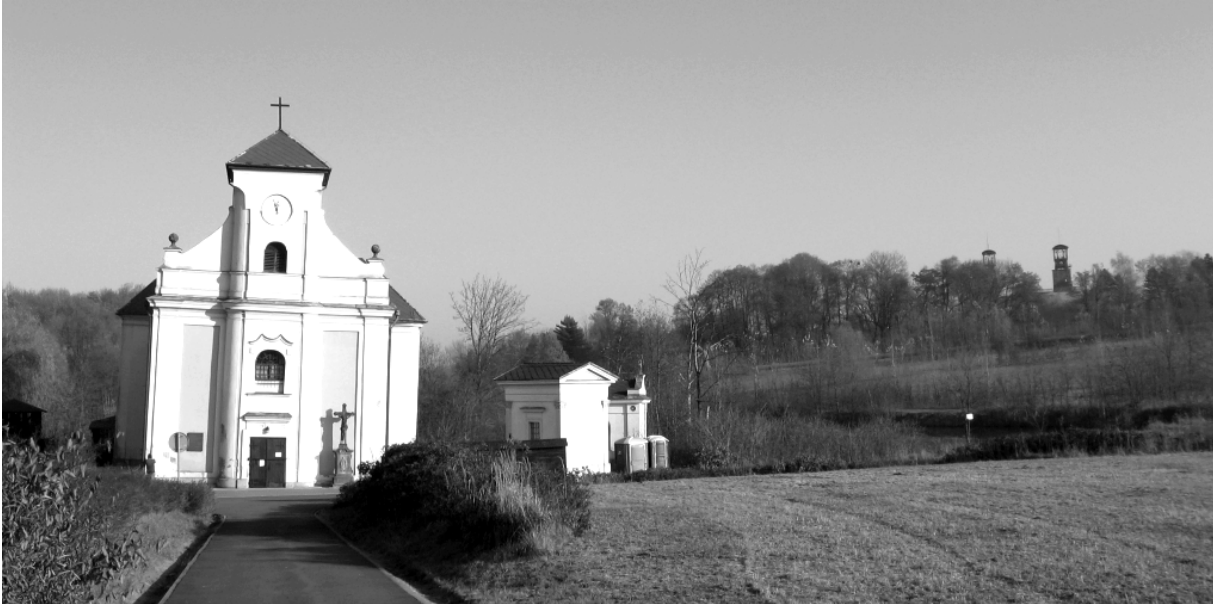
Fig. 1 The leaning Church of St. Peter of Alcantara and the Gabriela mine.
