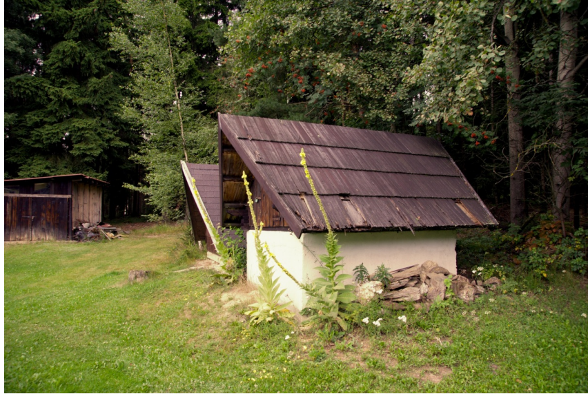
Fig. 2a Station Nový Kostel (NKC) – outdoor situation. The seismometers are situated in cca 5 m depth well, which is protected by “small chalet”.
