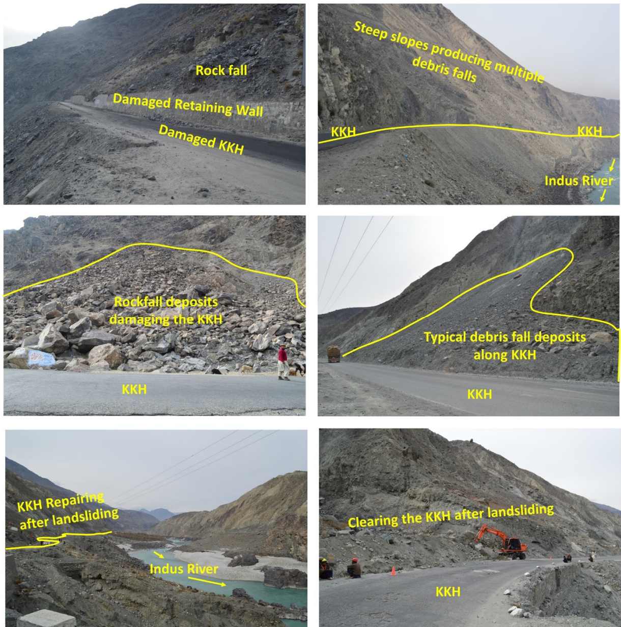
Fig. 3 Typical landslides in Dasu (Kohistan District) along KKH.
