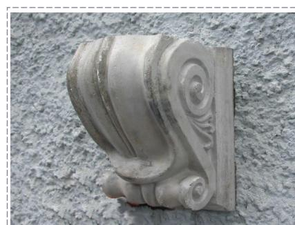
*Fig. 2: Architectural ornament: voluta made of a geopolymmer (archive of the IRSM)*
