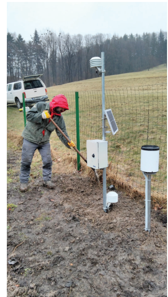
Installation of automatic climatic and environment monitoring station (CZ)
