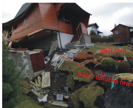
Poláky landslide: The scarp and damaged house at the village of Poláky landslide (2014, CZ)
