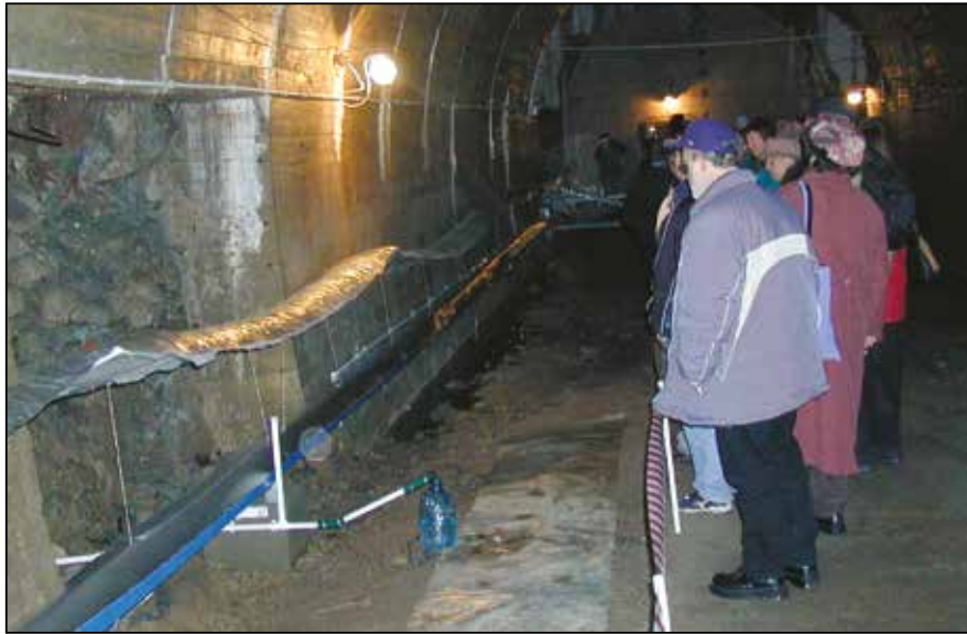
The Institute of Rock Structure and Mechanics is a co-organiser of Czech-Polish workshops. The 4 th workshop, held in Lubawka in 2002, included an excursion to the geodynamic laboratory under the Ksiaz chateau in Poland where the rock mass tilt is permanently monitored using a tube in the laboratory's long corridors. IRSM, Vladimír Schenk's personal archives.
