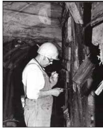
Robert Brož measuring fissures with a geological compass, Příbram Coal Mines, undated. Photo by Renáta Louvarová (Záběhlická). IRSM, collection of photographs.
