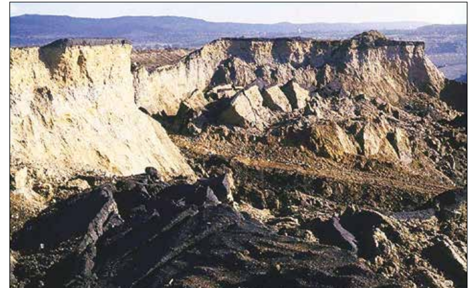
Deep slide affecting the overburden benches at the ČSA giant coal opencast; Krušné Mts. fault slope at the rear. Photo by unknown author.
